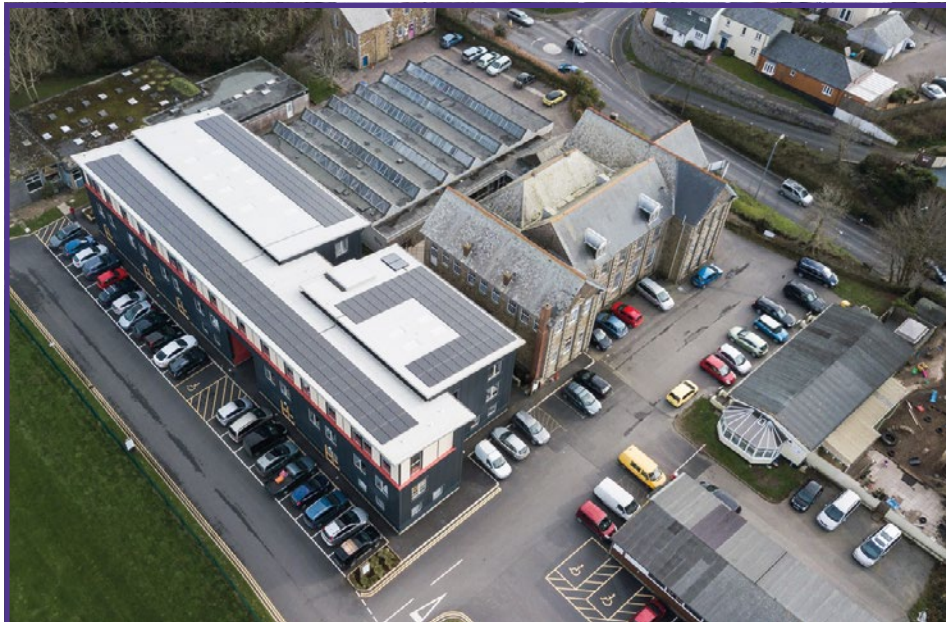
Creative Kernow Aerial shot post Phase 1. Photo © Luke Holland
